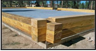
In **Muddy Cluster** the lodge being constructed on the Circle of Life property is moving forward as logs are milled. Rev. Dennis Bauer shared that the structure now has two or three beams on each side with electrical boxes for outlets in the beams.. Groups of workers from around the United States will volunteer their time this summer to work on this project and offer Vacation Bible School programs for the youth.
